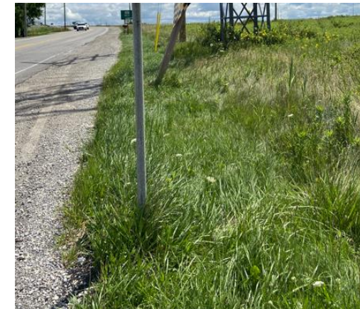
Ditch along Oxford Rd 15 (EBL)
