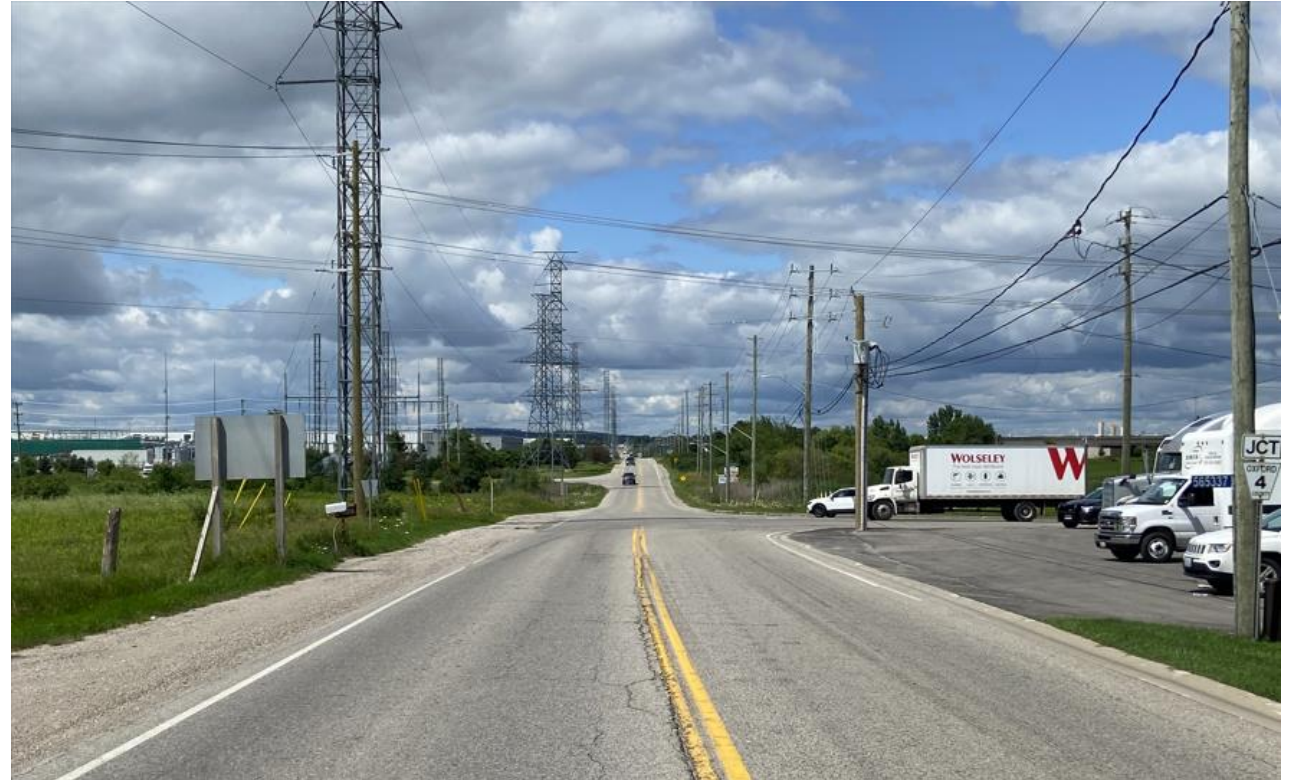
Existing hydro infrastructure
