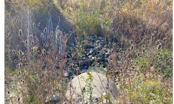
Culvert downstream toward pond
