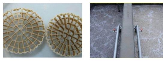
Figure 3.6 MBBR Media (left) and Reactor (right)
