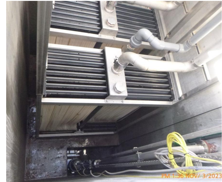
ZeeWeed 500D microfiltration membrane cassettes
