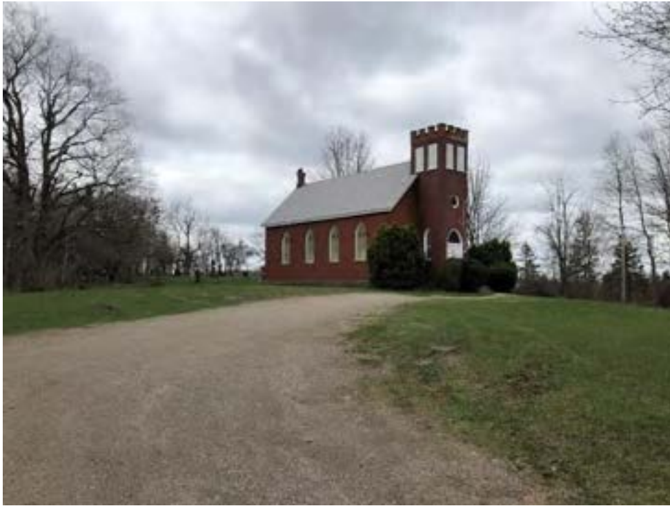
Image 12 St. Charles Anglican Church and Cemetery requires avoidance. Areas beyond disturbed path require Stage 2 survey
