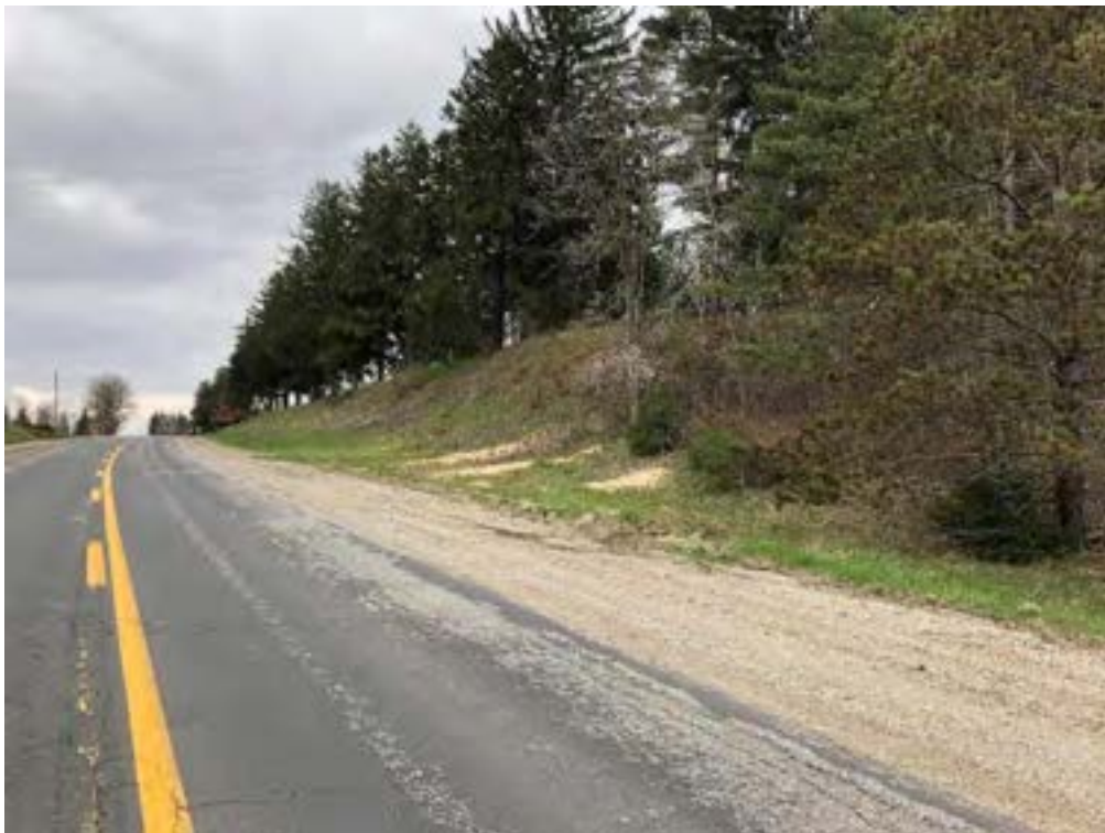
Image 33 Area beyond disturbed road cut requires construction monitoring
