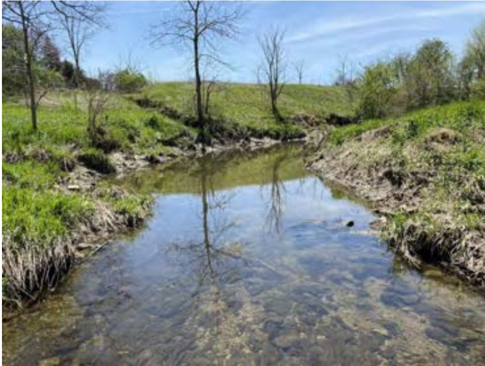
Photo 11 Looking south upstream from the inlet of the bridge.
