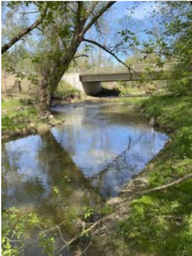
Photo 8 Looking north at the bridge downstream of the road
