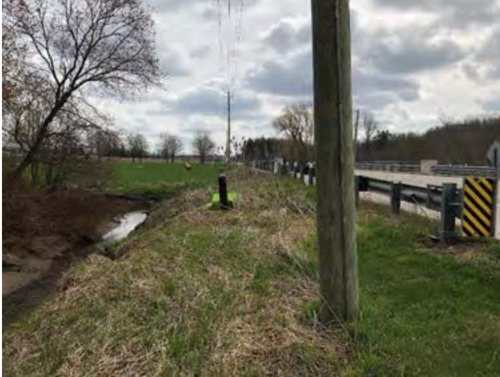
Image 7 Area beyond disturbed right-of-way requires Stage 2 survey
