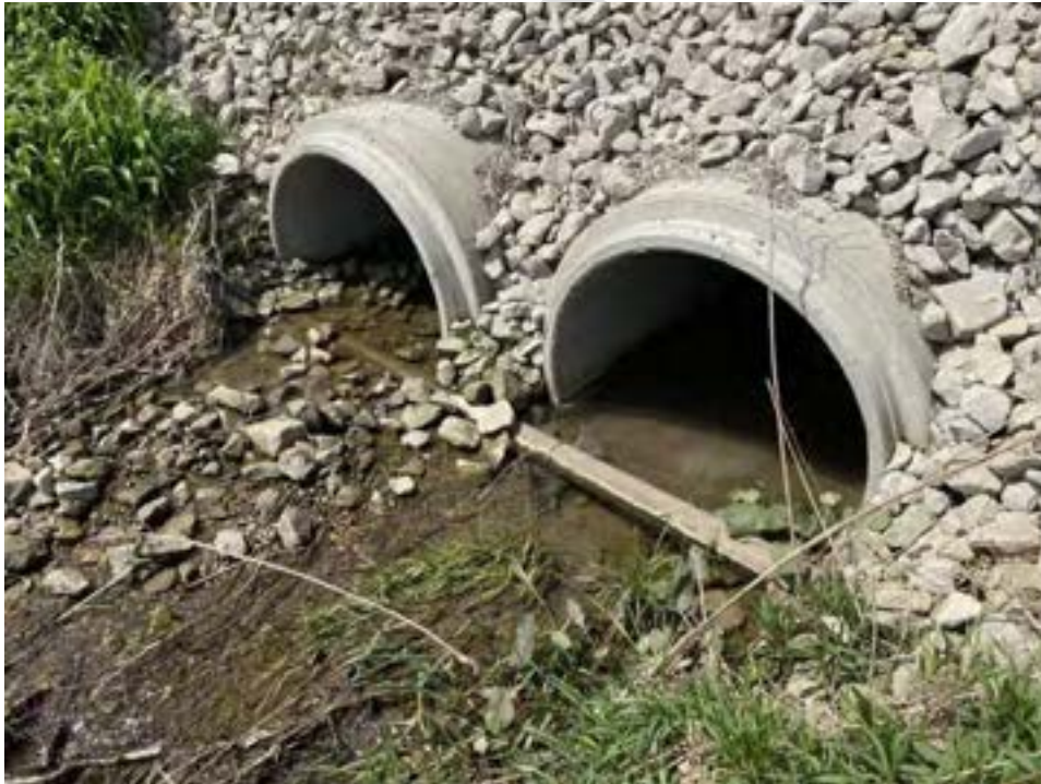
Photo 23 Looking down at the outlets of the culverts.
