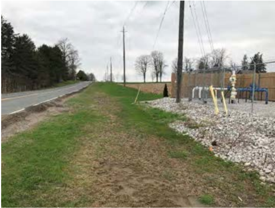
Image 54 Area beyond disturbed right-of-way and transformer station requires Stage 2 survey.
