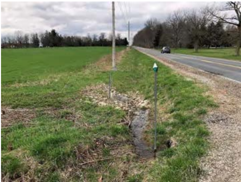
Image 13 Area beyond disturbed right-of-way requires Stage 2 survey
