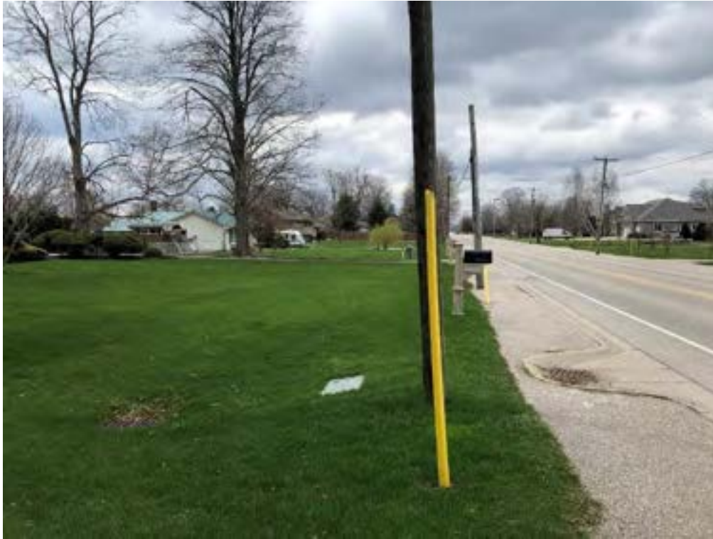
Image 24 Area beyond disturbed right-of-way requires Stage 2 survey
