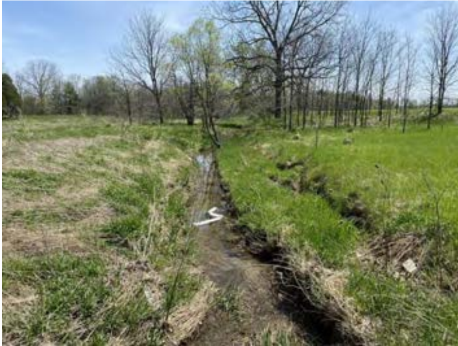
Photo 22 Looking south downstream from the outlet of the culvert
