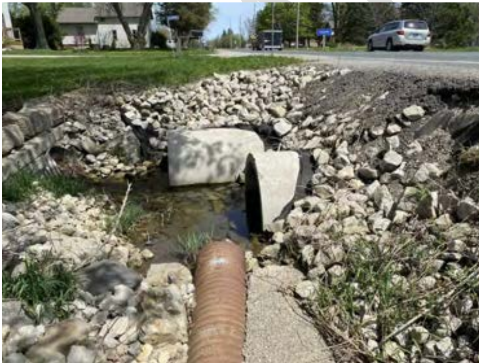
Photo 25 Looking down at the two tile outlets into the watercourse.
