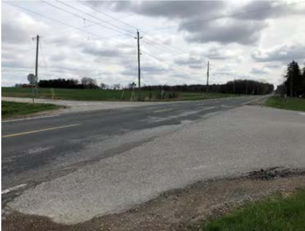
Image 9 Area beyond disturbed right-of-way requires Stage 2 survey
