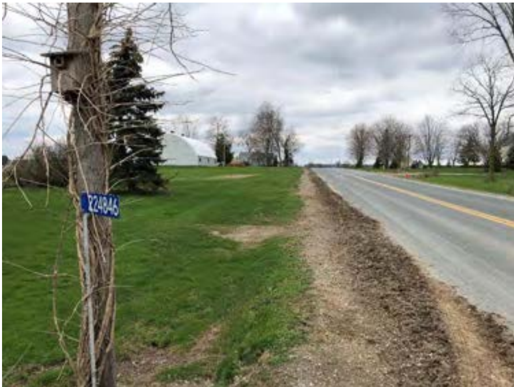
Image 19 Area beyond disturbed right-of-way requires Stage 2 survey
