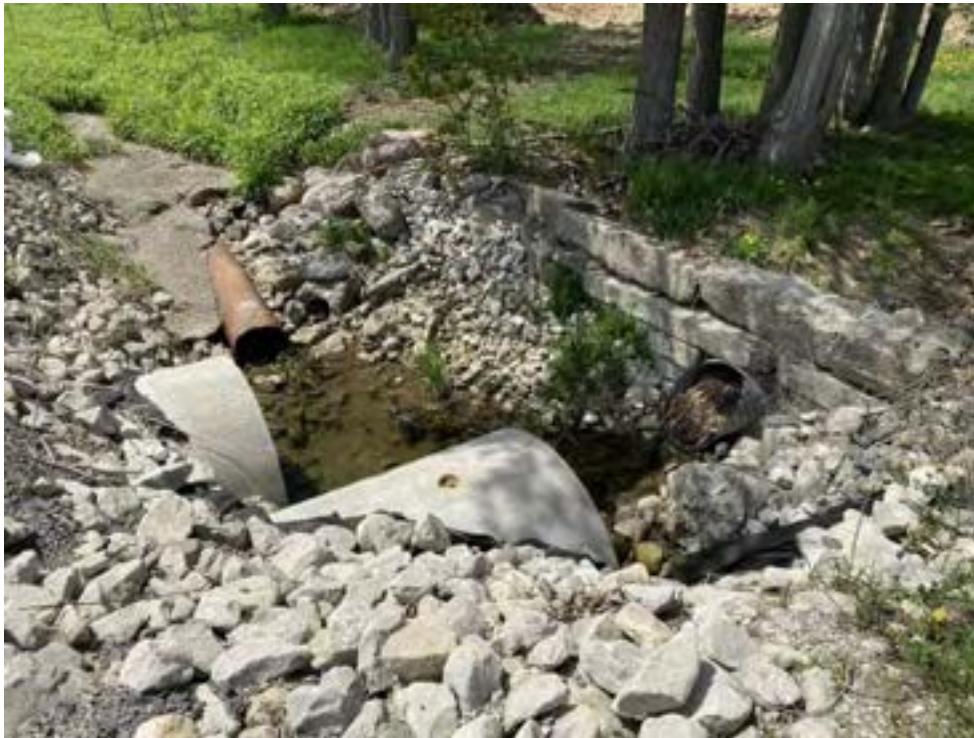
Photo 24 Looking down at the inlets of the culverts.
