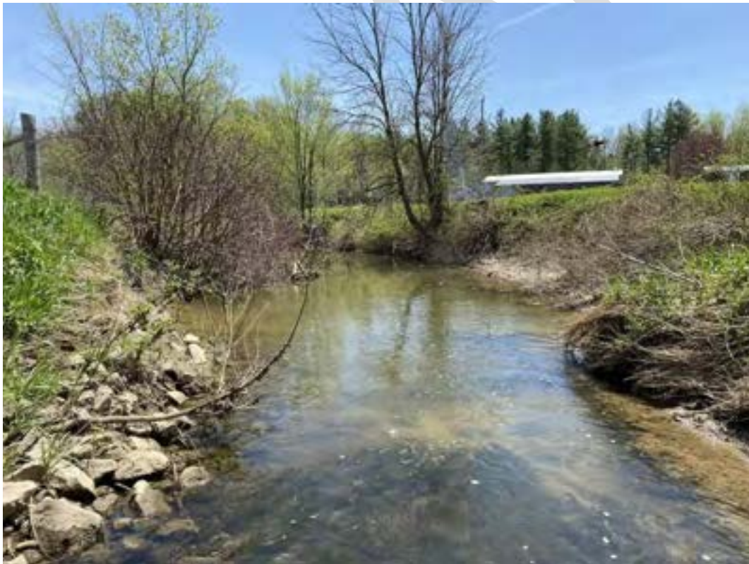
Photo 16 Looking southeast, downstream from the outlet of the bridge
