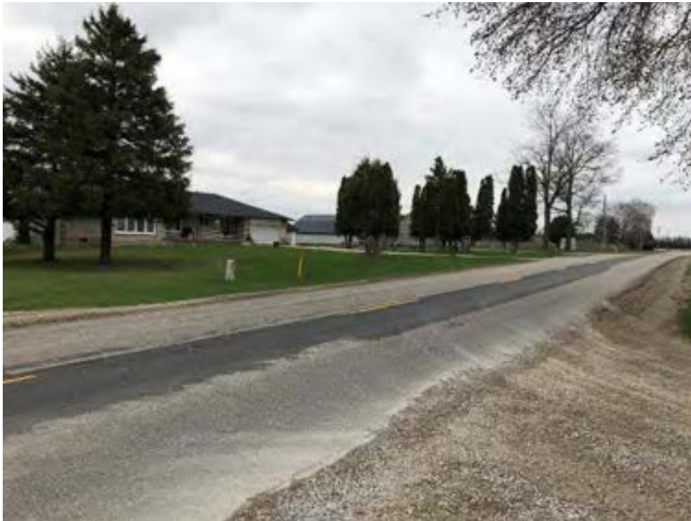
Image 49 Area beyond disturbed right-of-way requires Stage 2 survey
