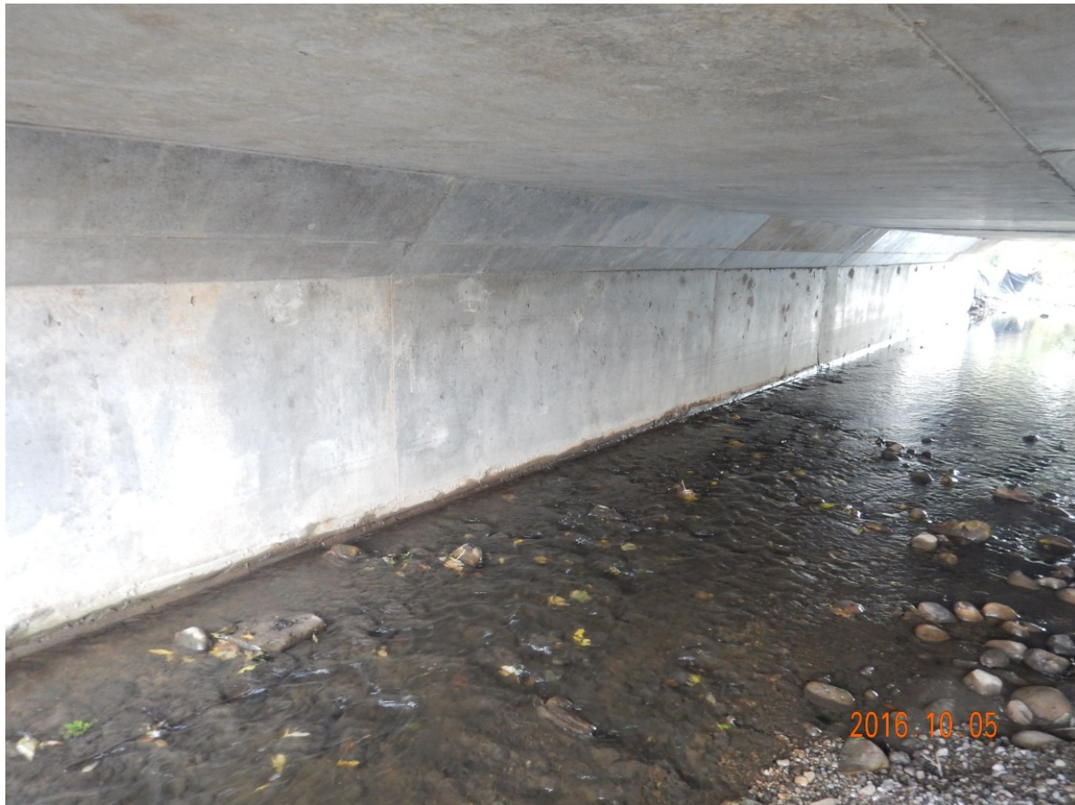
Image 4.0.1 Concrete Culvert with a BCI of 99.41 (Excellent)
