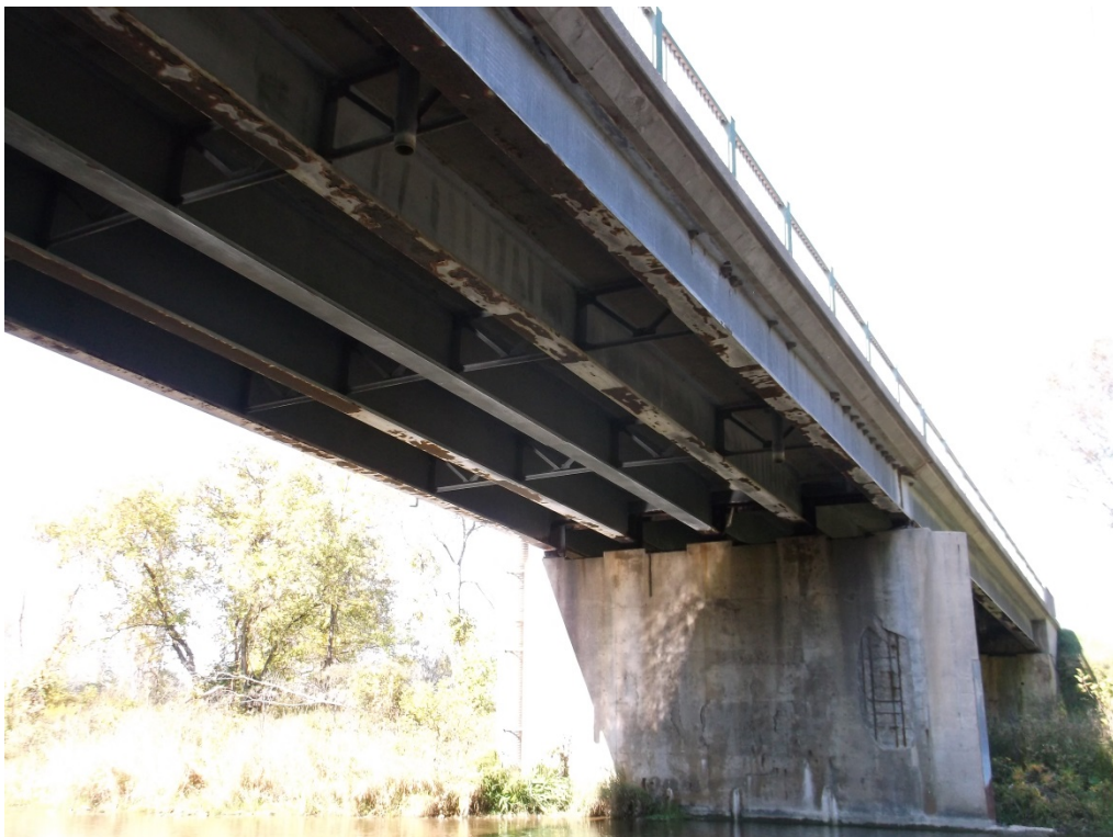
Image 4.0.3 Steel I-Beam Bridge with a BCI of 56.72 (Fair)
