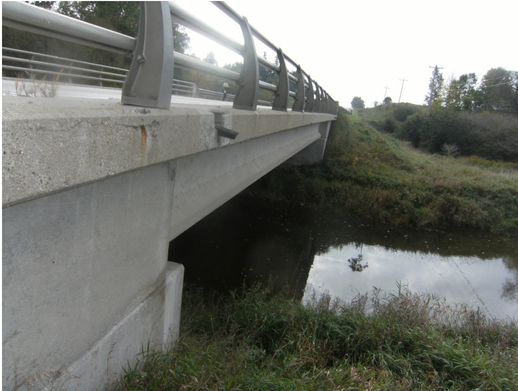
Image 4.0.3 Steel I-Beam Bridge with a BCI of 56.72 (Fair)
