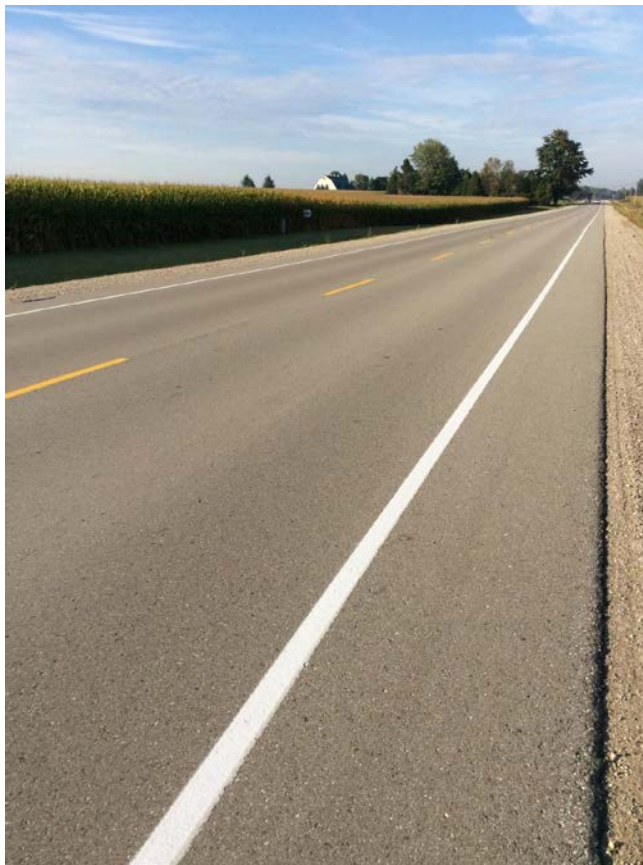
Image 4.0.1 Rural Road with a PCI of 92.9 (Excellent)
