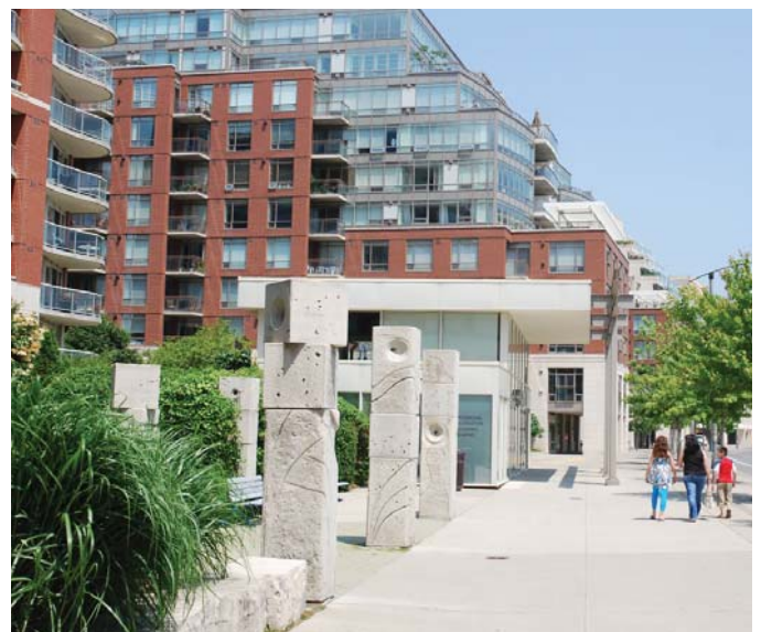
A portion of large developments can be setback to create urban plazas.
