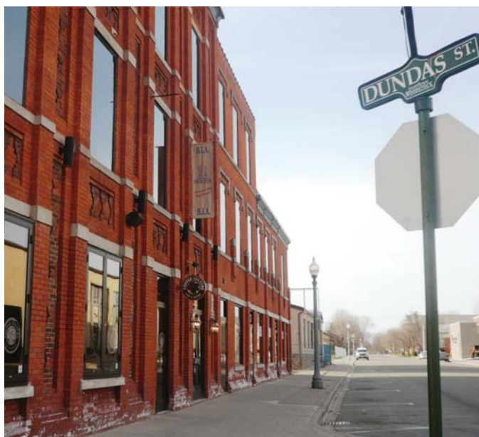
Graham Street near Dundas Street.
