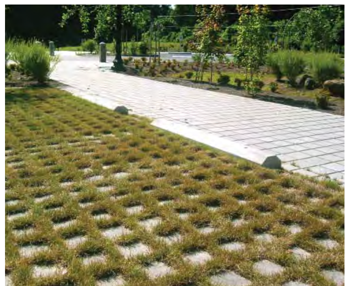
Porous pavement, and landscaped areas with adequate size and soil conditions, should be maximized.
