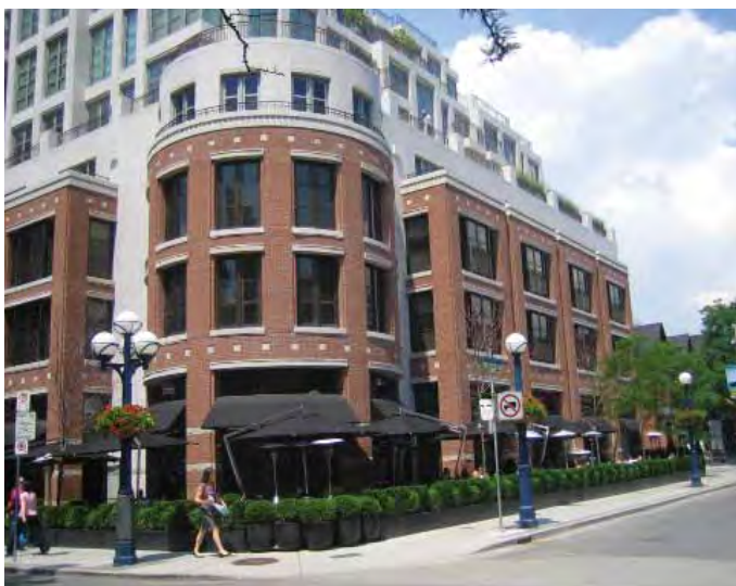
Windows in new buildings may be made of pre-finished metal or wood so long as proportions and configuration are maintained.
