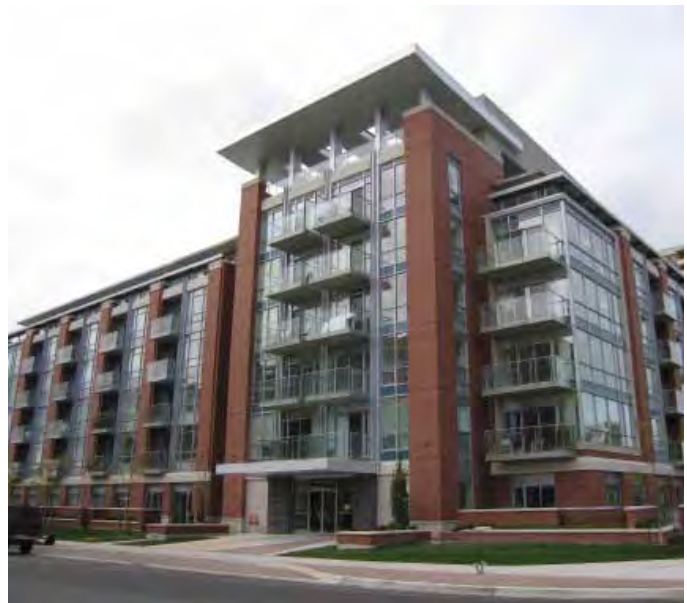
The redevelopment could take the form of a mid-rise building, with active uses along Broadway Street as well as along the edge of the parkette.
