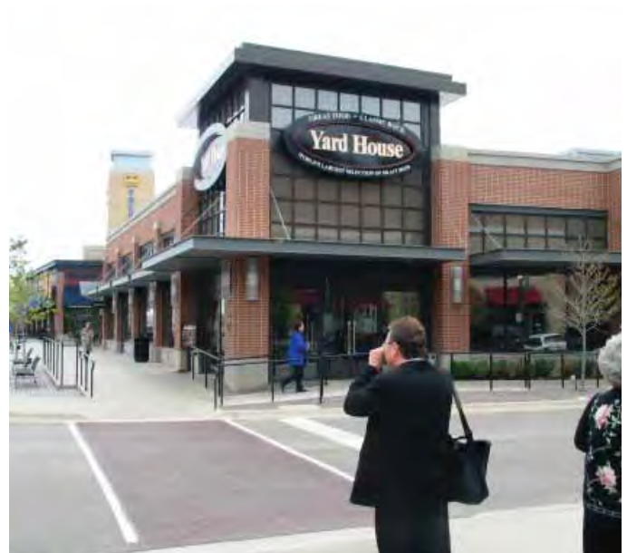
Strategic measures can more wholly integrate large buildings into the urban fabric of Tillsonburg's Central Area.
