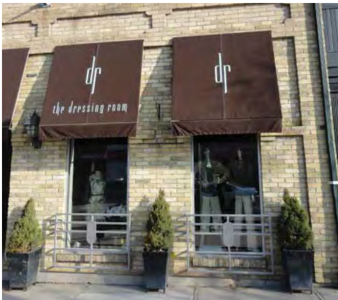
Awnings and canopies should be designed to match the main structural elements of the lower facade.
