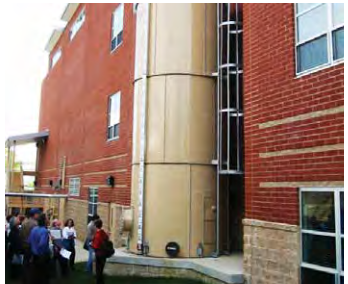
Waste water technologies, such as rain barrels or cisterns, are encouraged to collect and filter rain water to be recycled for non-potable domestic use.
