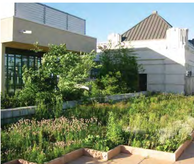
Vegatated or “green” roofs are recommended, especially in areas with minimal landscaping.
