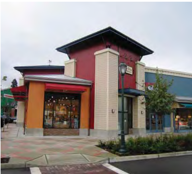
The principle building entrance should be highly visible with features such as canopies or porticos, arcades and landscaping.
