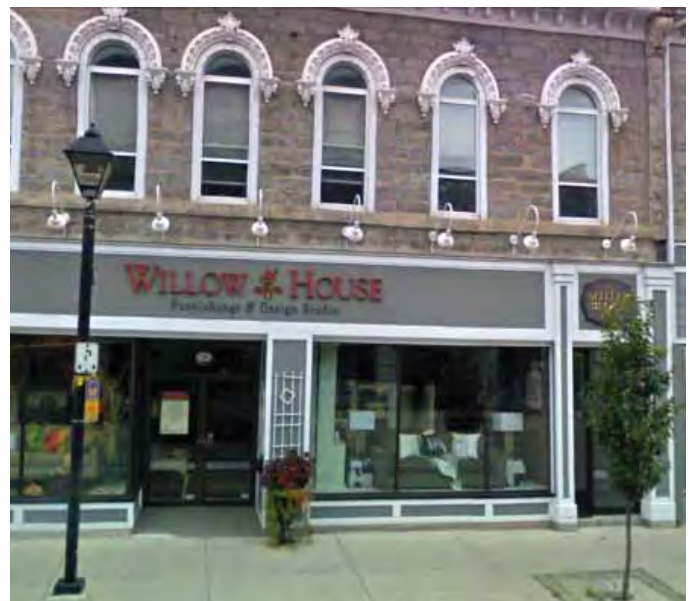
Fixtures may be chosen from available replica styles appropriate to the architecture of the heritage buildings.
