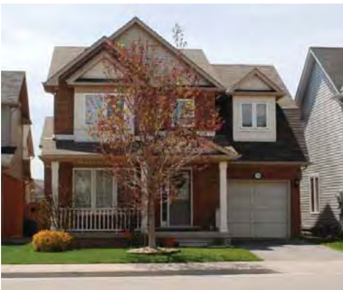
Driveways should be no wider than the width of the garage, which should be limited to 50% of the width of the dwelling.
