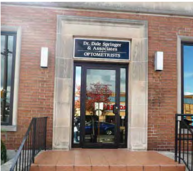
Spalled stonework can be restored using professional epoxy-based fillers.
