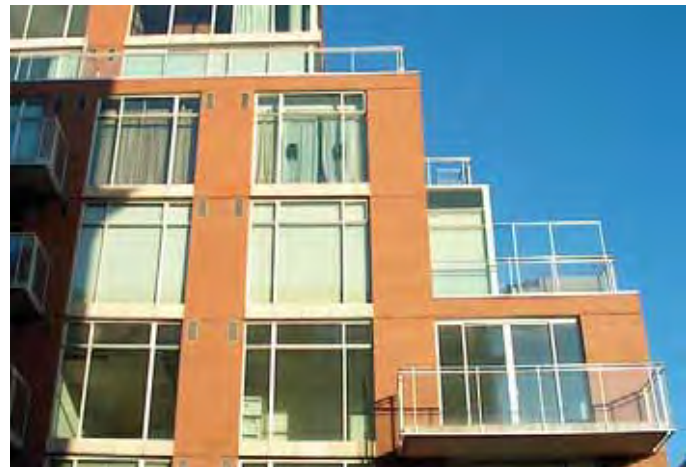
Stepbacks should be provided above the 3rd storey to maintain an appropriate sense of scale from the street.
