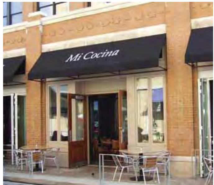
Awnings and canopies should be designed to match the main structural elements of the lower façade.
