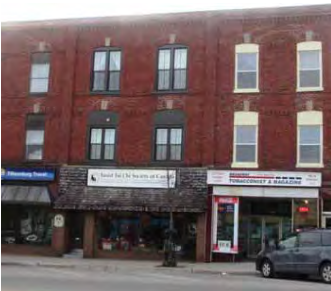
Original windows and doors should be repaired if possible.
