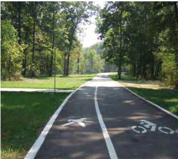
The design of multi-use trails should distinguish between walking and cycling areas to minimize conflicts.
