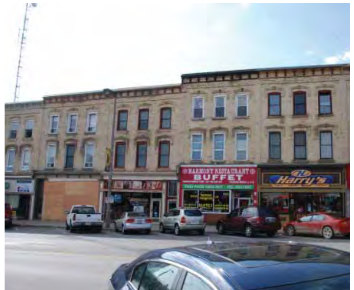
Like much of Southwestern Ontario, Tillsonburg's Central Area contains an abundance of historic yellow brick buildings.
