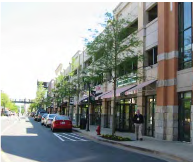
Structured parking should be developed with active at-grade uses to provide attractive facades, animate the streetscape and enhance pedestrian safety.
